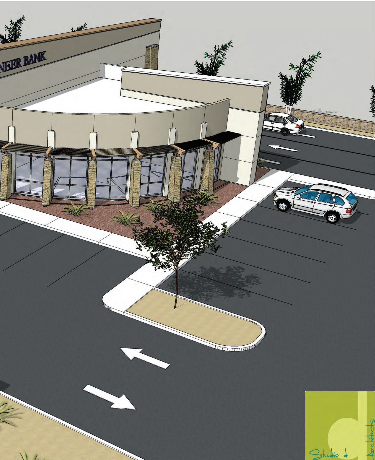
Pkwy, Las Cruces, New Mexico. Construction to be completed by November 2021.
